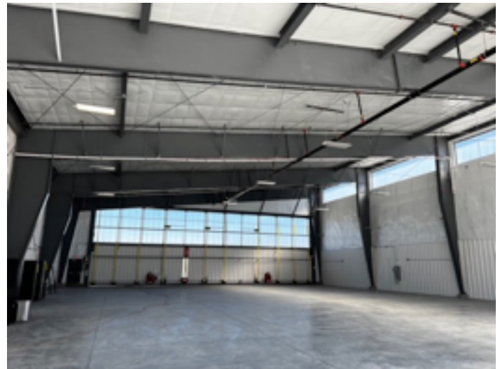
One of the new hangars awaits its first occupants.
