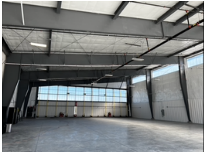
Many of the hangars are "pull through" with doors which open on both ends.
